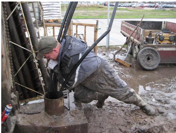
Installation of borehole heat exchanger at test site, photo Inga Sørensen VIA UC.
