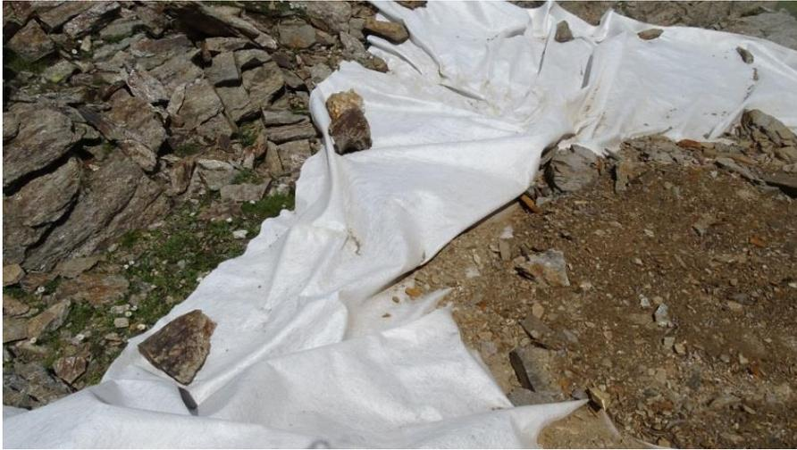
Figure 3: Protection of a snowbed area through a geotextile and a layer of mineral soil rich in stones
