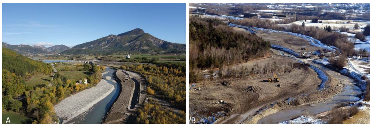
Figure 1. Emblematic recent sediment replenishment operations in French alpine gravel-bed rivers: (A) sediment replenishment downstream of the Saint-Sauveur dam in the Buëch River in 2016 (@EDF); (B) sediment replenishment of the incised Upper-Drac River in 2014 (@CLEDA)
