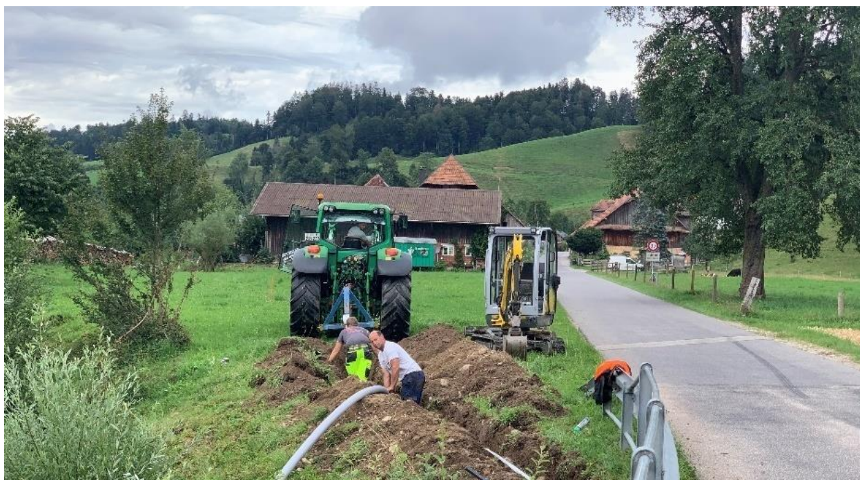
Figure 8. The local fibre optic network of Luthern being installed (RLW)
