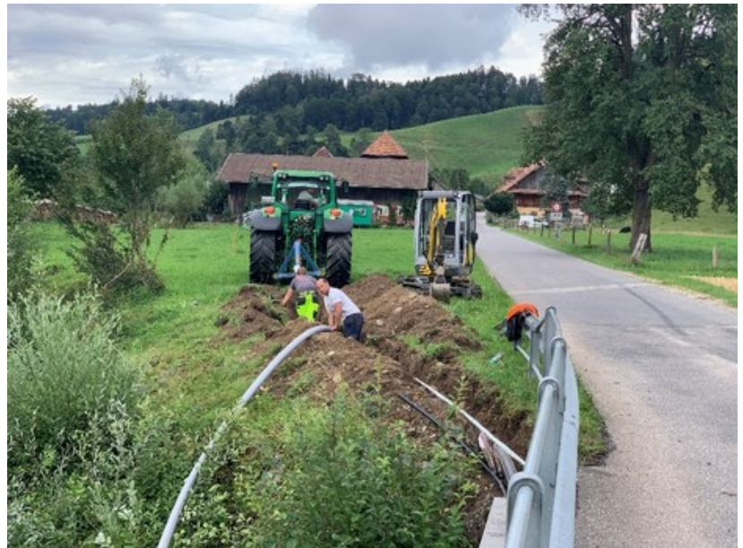
Figure 7: The local optical fibre network of Luthern is being installed
