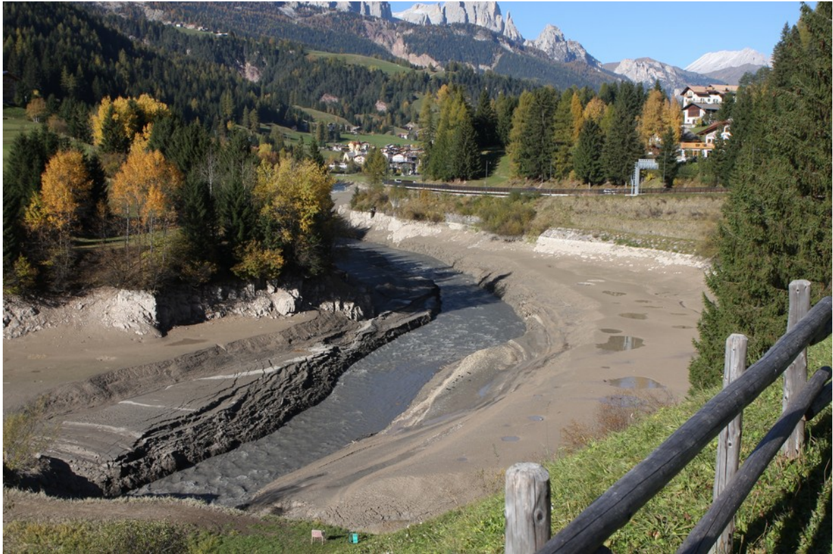
Figure. 4: The Pezzè reservoir during sediment flushing operations.
