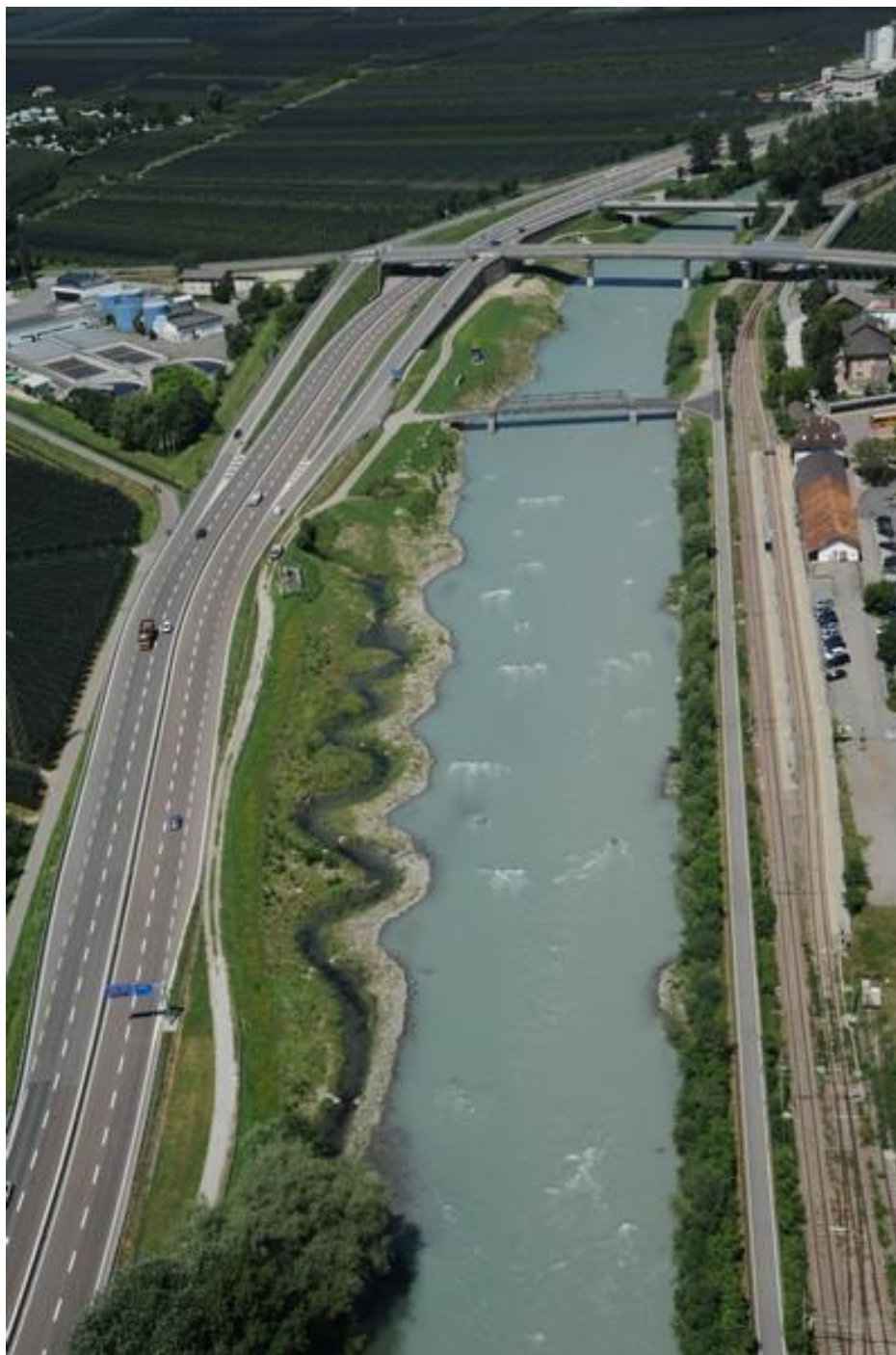
Figure 4 - Restoration works along the orographic right of the Adige River (2012). Inlets along the reach and boulders distribution on the riverbed. Connection of the lateral ditch with the Adige favoring fish passage and habitat
