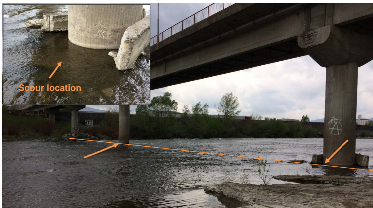
Figure 14. Area of interest 2 – bridge column scour locations (arrows)
