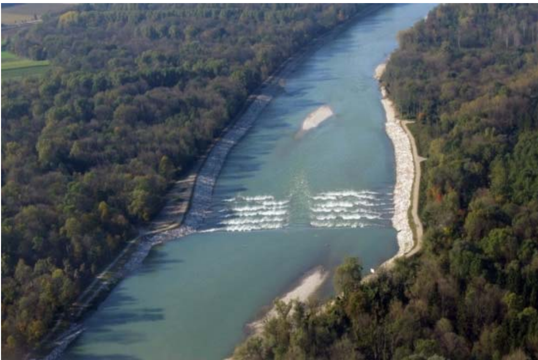
Figure 5. Step-pool ramp constructed in the year 2010 in the Salzach River to rise the bed level upstream. Removal of bank protection downstream intended to compensate the bedload deficit which resulted from sediment trapping upstream of the reservoir.
