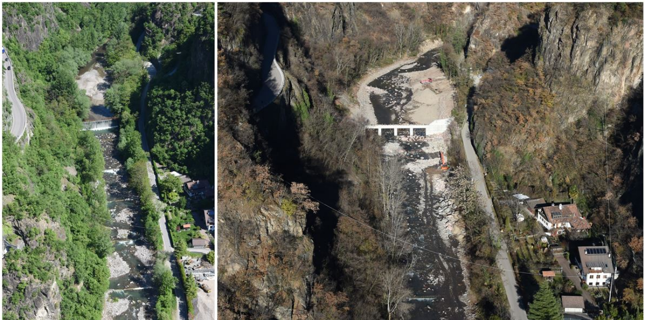
Figure 4: Consolidation check dam previously on site (left) and lately substituted by a retention check dam (right)
