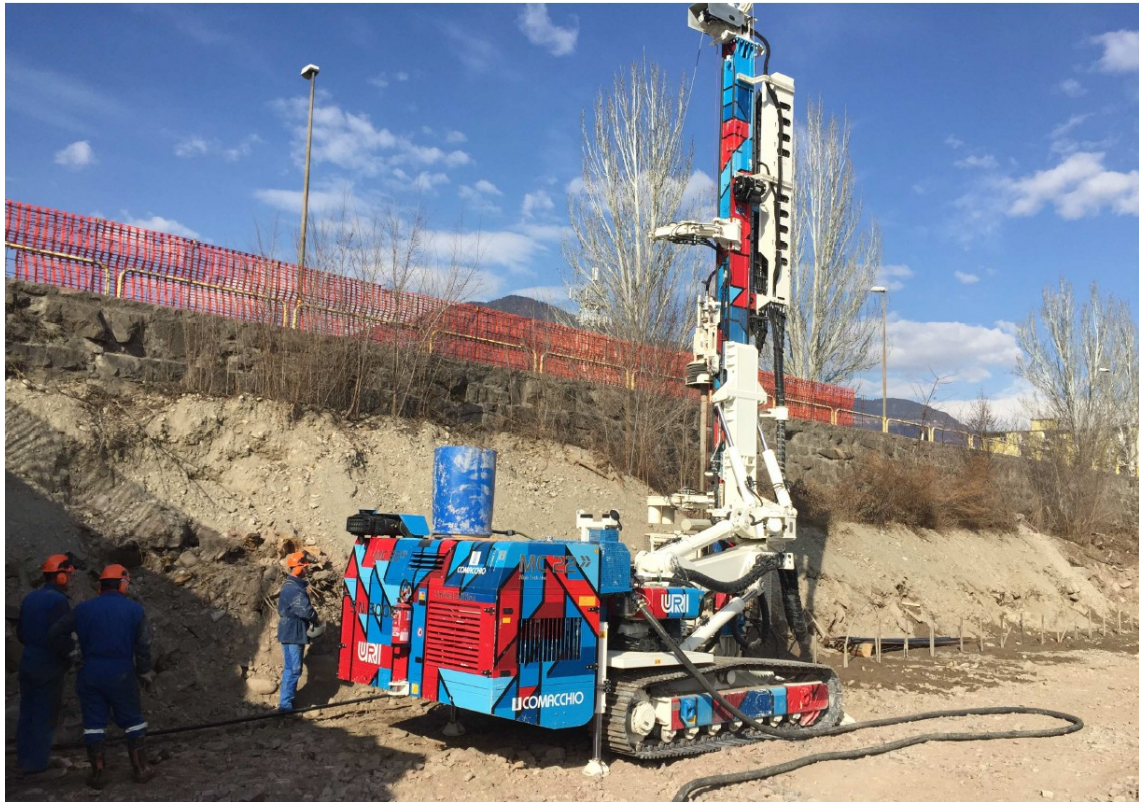
Figure 2: Construction of micropile bulkhead and reinforced concrete kerb to support the bank defences
