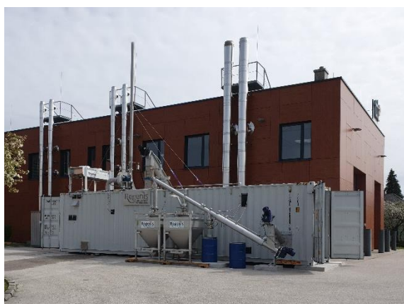
Figure 7: left: Pilot Scale pyrolysis plant from outside; right: pyrolysis plant inside container, pyrolysis reactor on left and gas burner on right side
