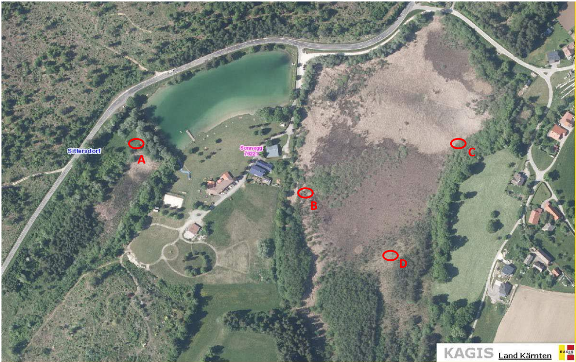
Figure 1.6: Establishment of spawning ponds for amphibians. Construction of amphibian ponds, place options A, B, C and D
