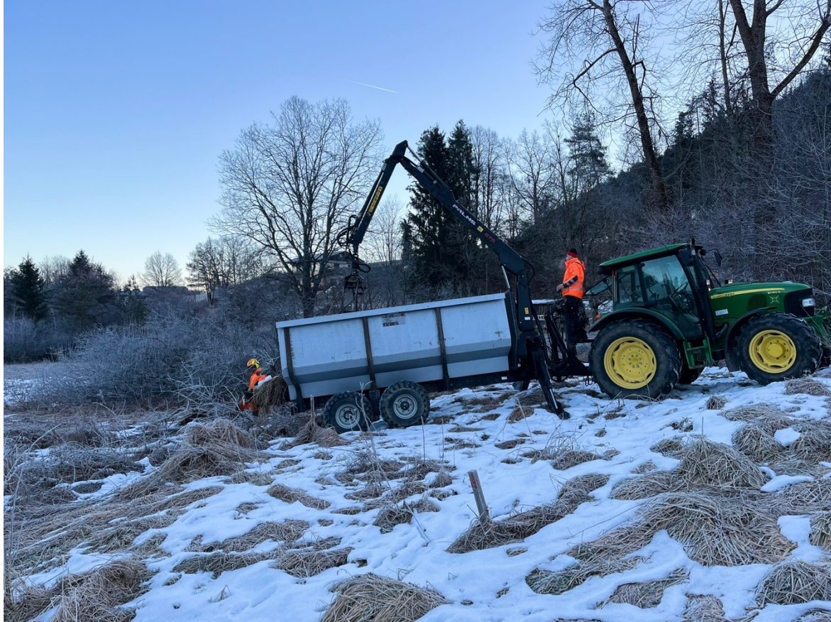
Figure 3.9: Access to peatlands with heavy machinery for the removal of trees and shrubs is advisable only if the ground is frozen (Sittersdorf, Austria, photo: S. Glatz-Jorde)
