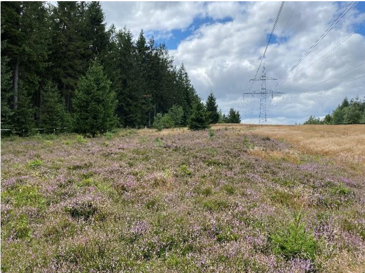
Figure 7: Example for heathland vegetation in the right-of-way of a 380 kV-transmission line
