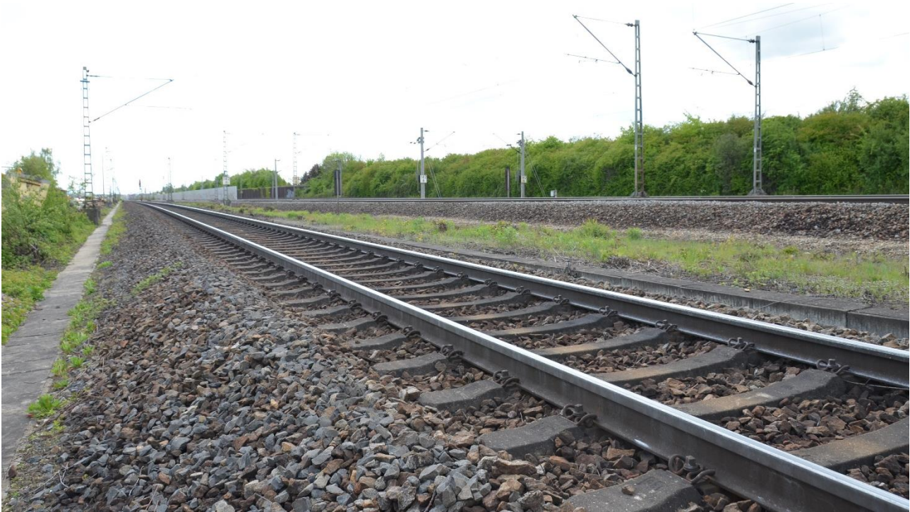
Figure 13: Railway: track bed with sleepers and rails
