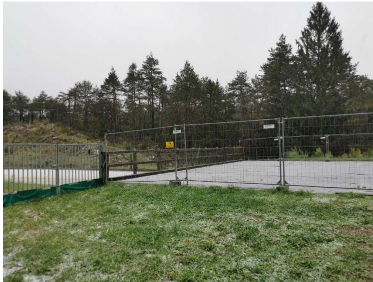
Figure 16: Gail outlet channel with fences as barriers
