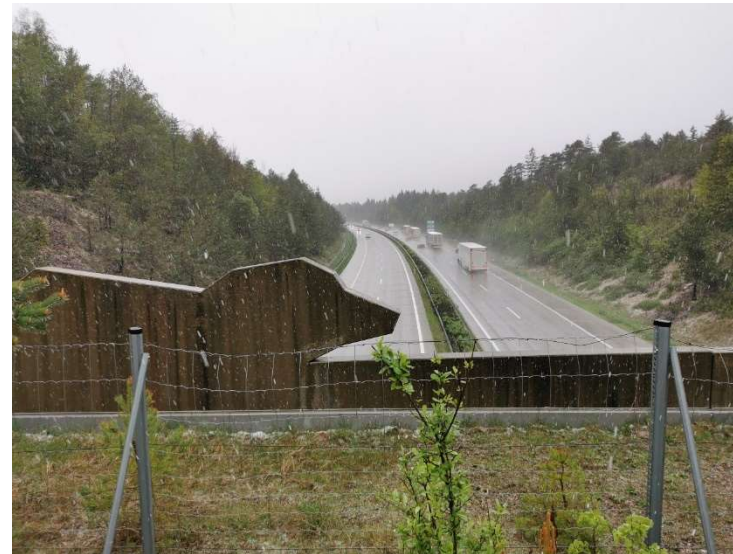
Figure 17: Bear bridge as connectivity element in the study area
