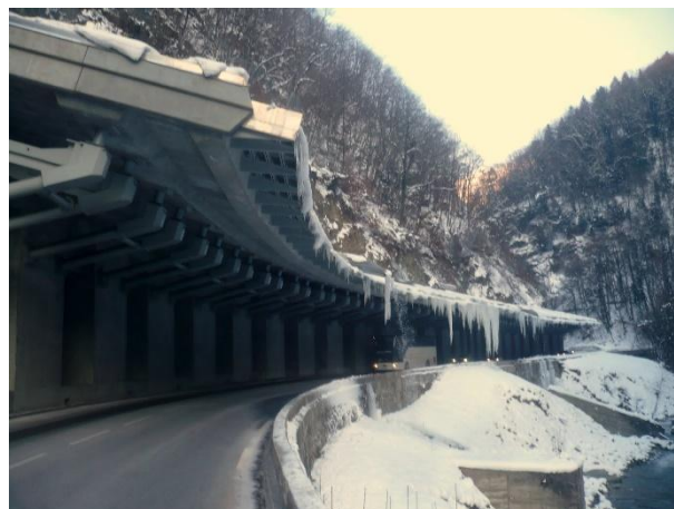
Figure 72 - Combe Noire avalanche defence structure, Arly gorges.
