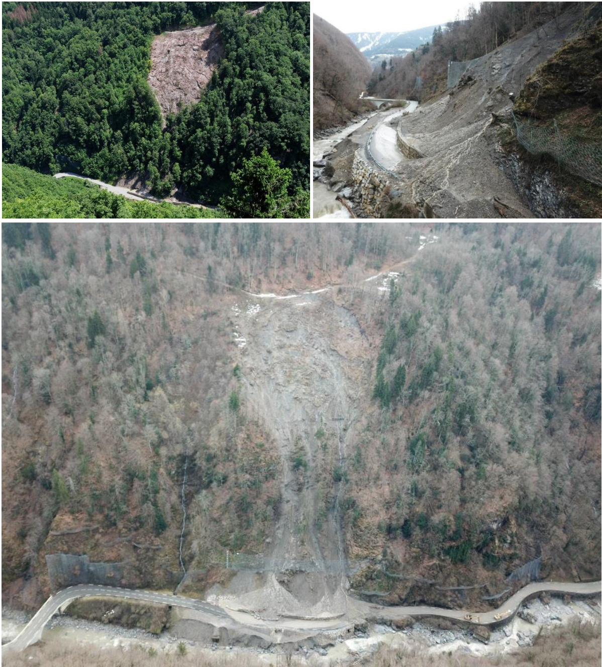
Figure 18 - Montgobert landslide, cutting the RD1212 after storm Eleanor in January 2018 (©Département de la Savoie).
