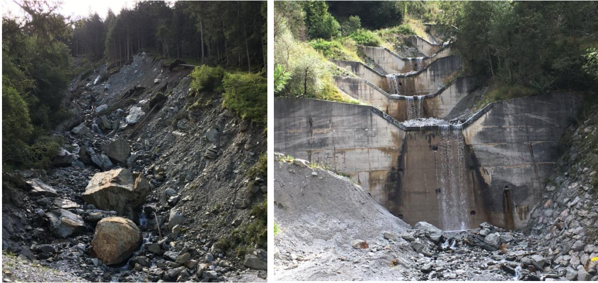
Figure 13: Debris flow channel of the Margaretenbach above the mitigation measures, showing the loose material source and large boulders - the biggest block has about 20 m 3 (left); mitigation measures in the Margaretenbach (right) (source BFW).
