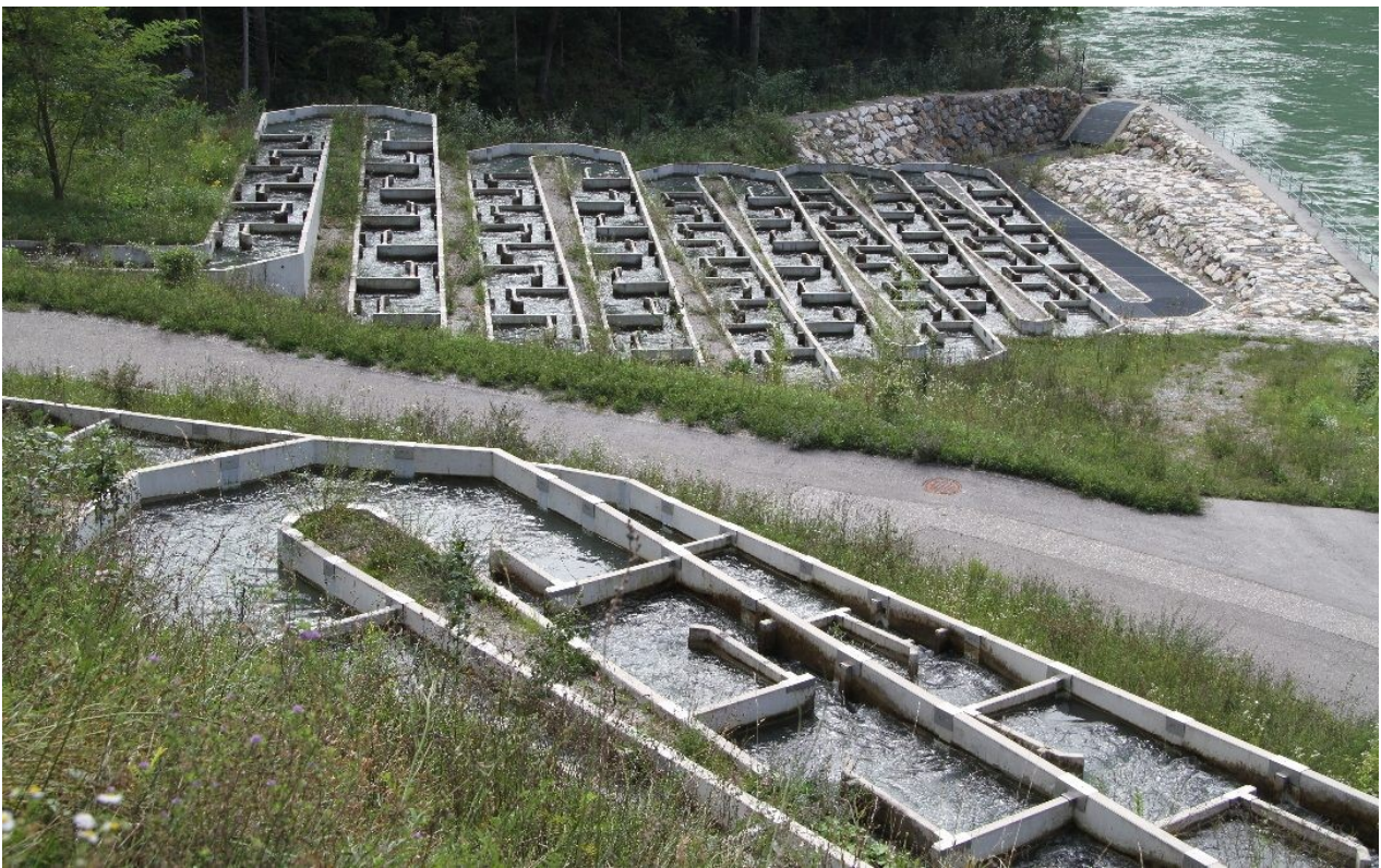
Figure 7: Fish ladder at Drau River (Example at Annabrücke). © Verbund 2024
