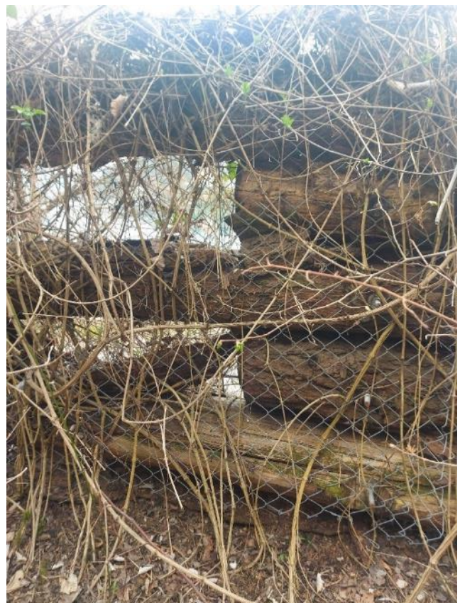
Figure 17: Temporary barrier consisting of 3 meters-high larch tree piles anchored into the ground, photo: Slovenia Forest Service
