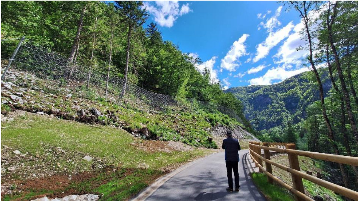
Figure 14: Rockfall protection barriers above the cycling path in Soteska, photo: Magdalena Cholkova
