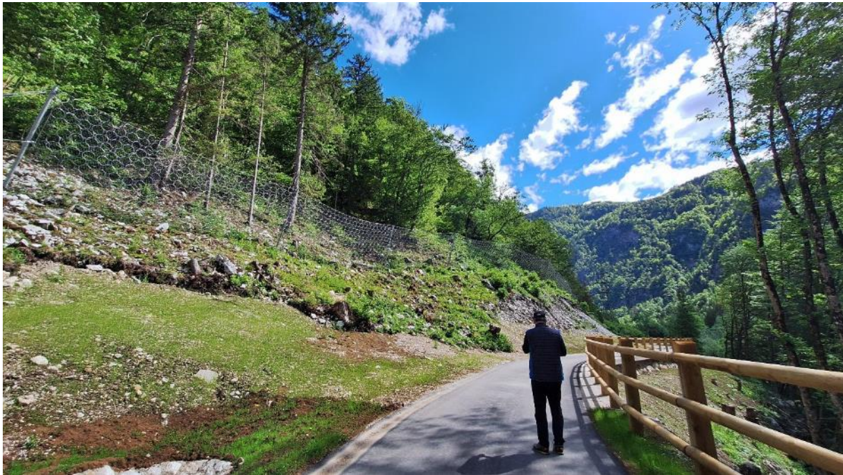
Figure 14: Rockfall protection barriers above the cycling path in Soteska, photo: Magdalena Cholkova
