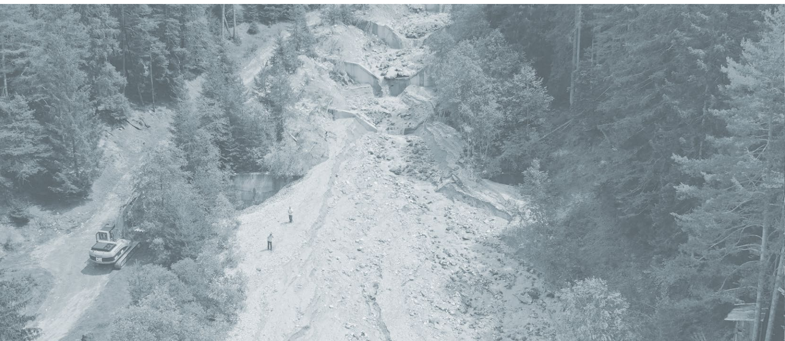
Damaged series of checkdams after the debris flow event in July 2022 on Margaretenbach in Fulpmes (Source: BFV Kufstein).
