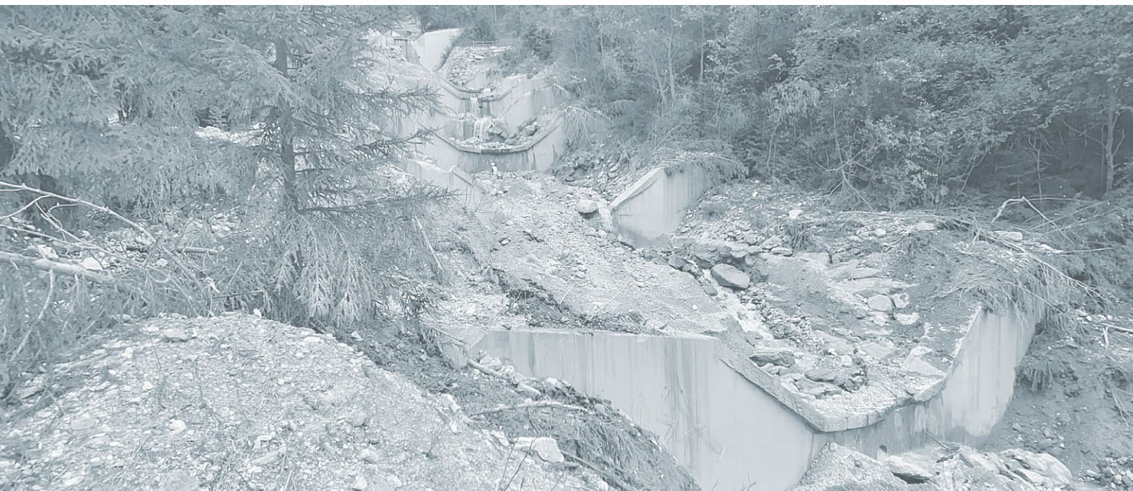
Damaged series of checkdams after the debris flow event in July 2022 on Margaretenbach in Fulpmes (Source: WLV).
