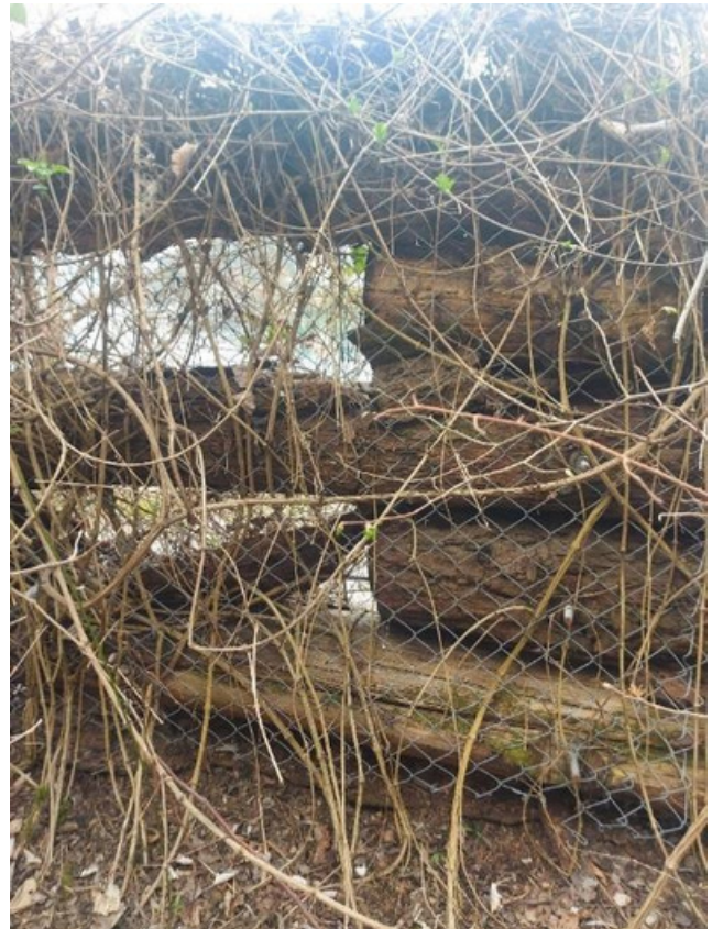
Figure 20: Temporary barrier consisting of 3 meters-high larch tree piles anchored into the ground, photo: Slovenian Forest Service
